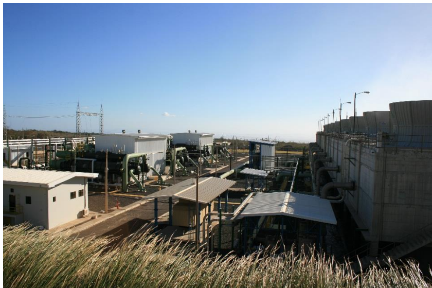
FIGURE 3: The Las Pailas binary geothermal power plant in Costa Rica
