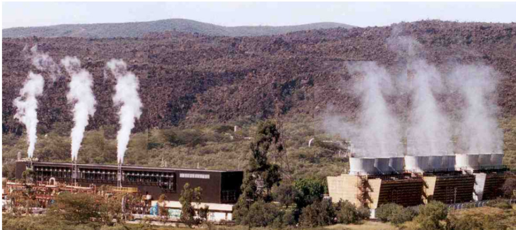
FIGURE 2: Olkaria I Power Station (45 MW)
