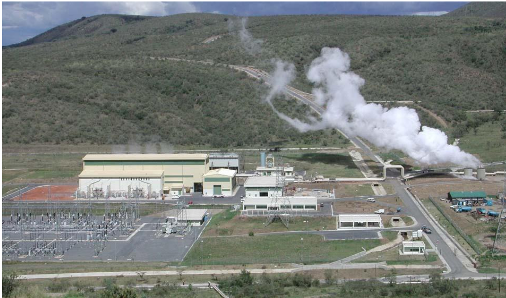
FIGURE 5: Olkaria II power station, commissioned in 2003
