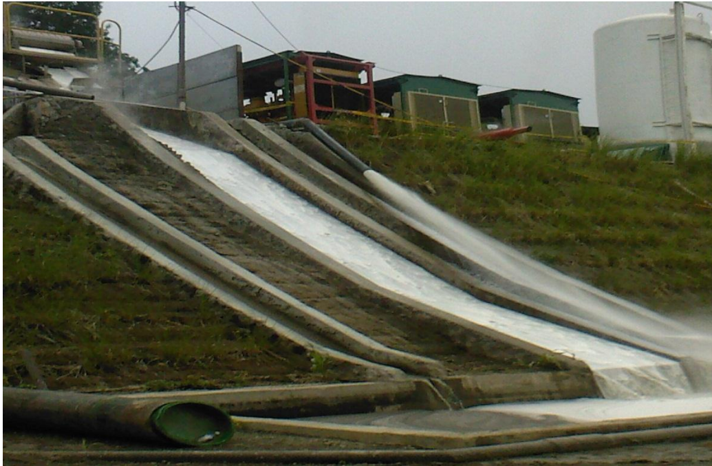
FIGURE 4: Return of the mixture water-air-foam-cuttings on the surface
