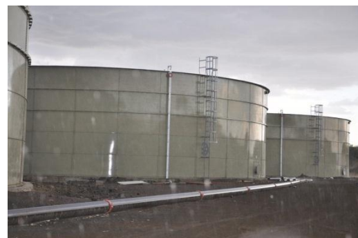
FIGURE 4: Water reservoir tanks at Menengai
