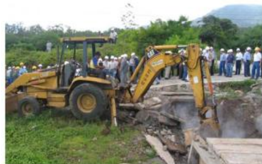
FIGURE 6: Decommissioning of the canal to the sea in August 2004
