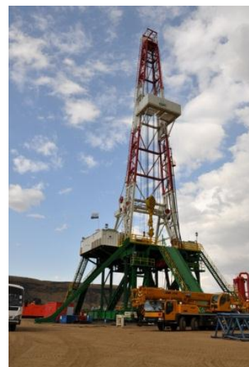
FIGURE 5: One of the new GDC 2000hp rig
