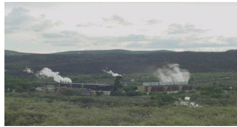
FIGURE 2: 45MWe Olkaria I Power station
