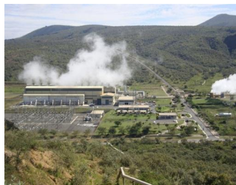
FIGURE 3: 105 MWe Olkaria II Power station
