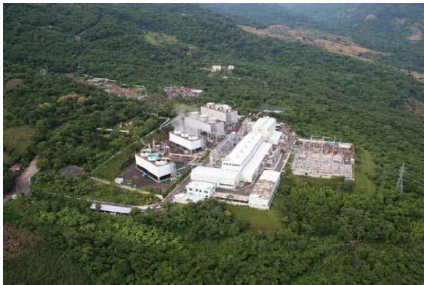
FIGURE 2: The Berlín geothermal power plant in El Salvador (Henriquez, 2008)
