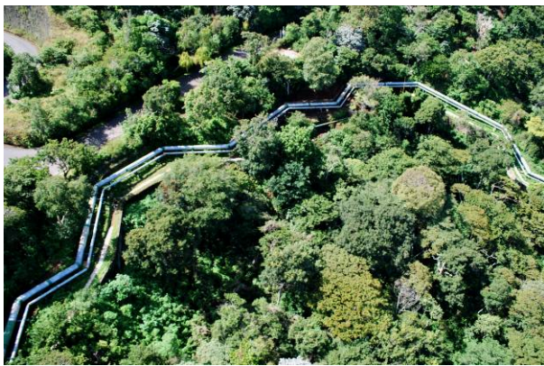
FIGURE 5: V Bend expansion loop
