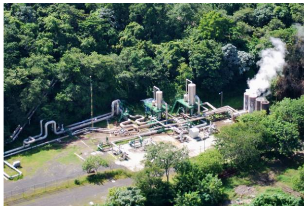
FIGURE 6: Omega bend expansion loop
