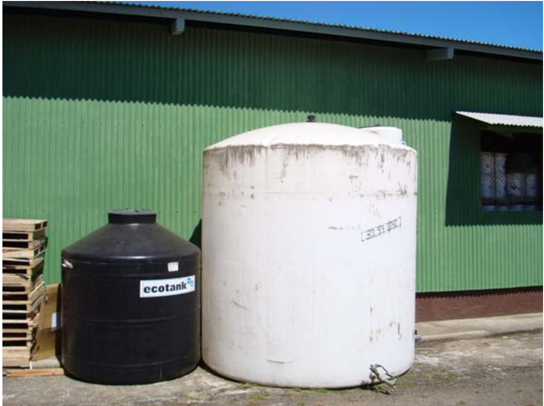
FIGURE 6: Inhibitor storage tanks (Photo by P. Moya)
