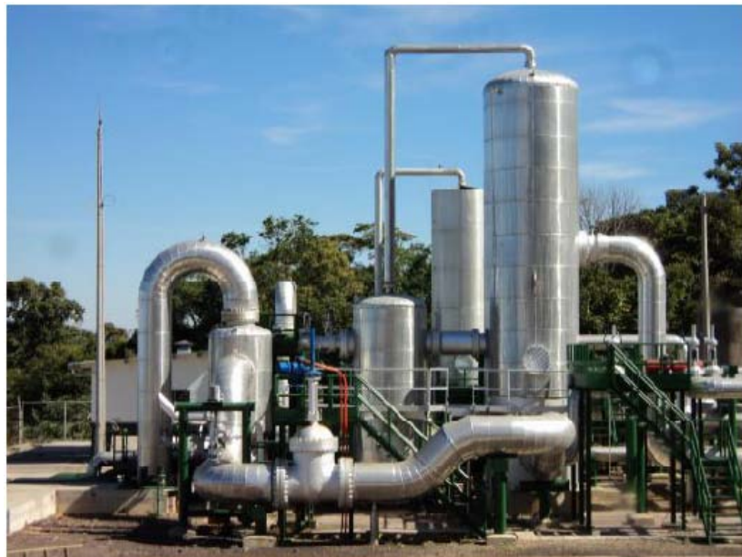
FIGURE 6: Separation stations in the same pad of TR-17 wells, Berlin geothermal field
