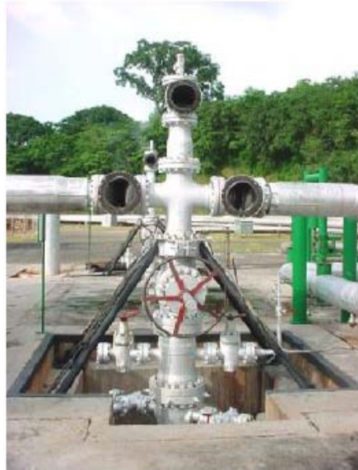
FIGURE 7: Disassembly of a production well wellhead valves for maintenance
