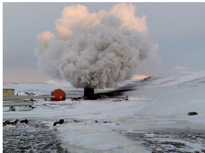
FIGURE 10: Well KJ-36 blowing (From: Thorhallsson et al., 2008)
