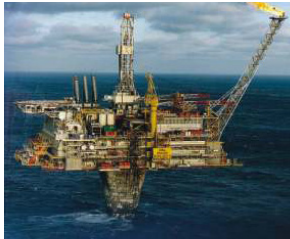
FIGURE 18: Jack-up marine rig
