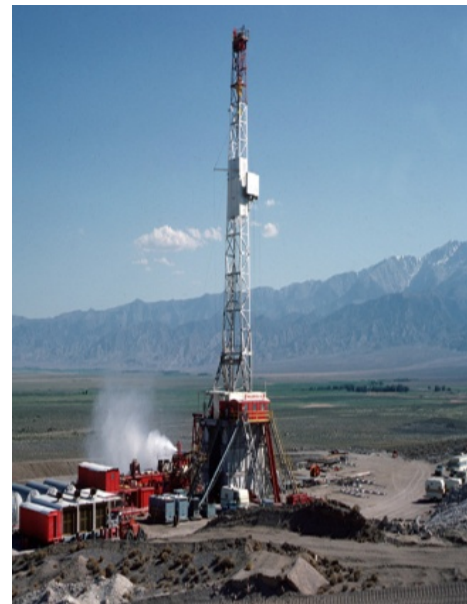
FIGURE 20: Typical conventional rig
