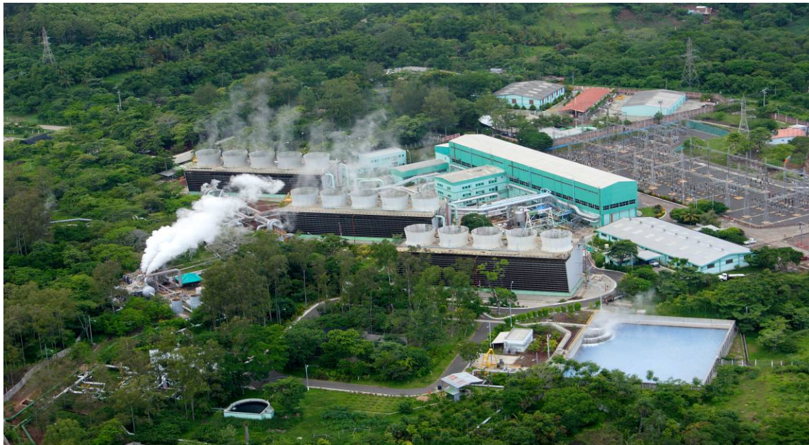
FIGURE 3: Aerial view of the Ahuachapán geothermal power plant
