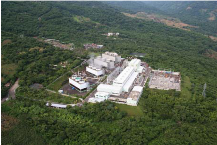
FIGURE 3: The Berlín geothermal power plant (Henriquez, 2008)
