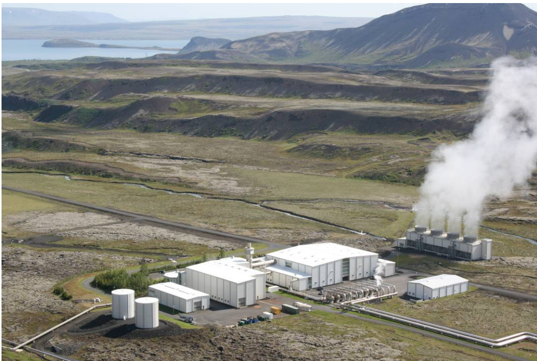
FIGURE 6: The Nesjavellir power plant in SW-Iceland produces now 120 MWe and hot water amounting to 300 MWth; the photo was taken in 2008
