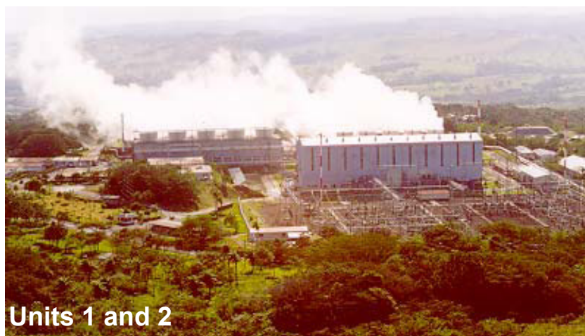
FIGURE 4: The Miravalles geothermal power plant (Vallejos-Ruiz, O., 2006)
