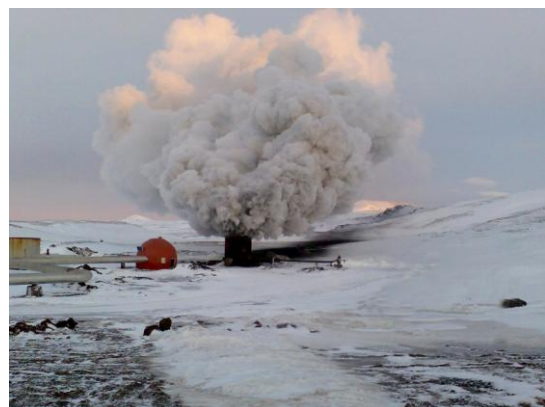
FIGURE 10: Well KJ-36 blowing (From: Thorhallsson, et al., 2008)
