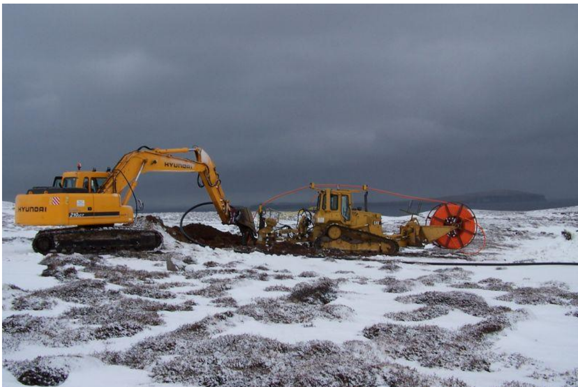
FIGURE 16: Installing the district heating pipe and fibre optic in winter.
