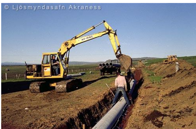
FIGURE 10: The asbestos cement pipes being laid into ground, un-insulated.
