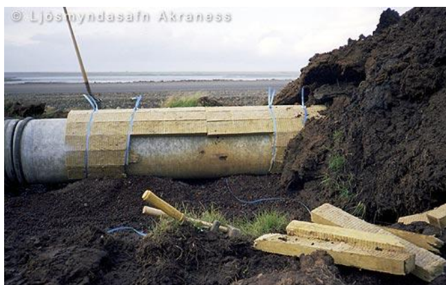
FIGURE 9: The asbestos cement pipes being laid above ground, insulated.
