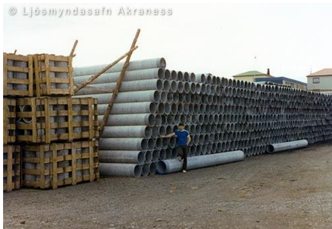
FIGURE 8: The asbestos cement pipes on the harbour in Akranes before the construction started.
