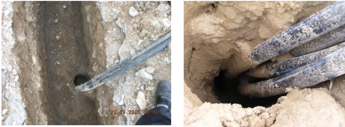
FIGURE 6: Single and double U-tubes for closed loop GHP (from Wang et al., 2008)
