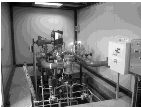
FIGURE 13: Well head installation of the combined production/injection well N 1/88
