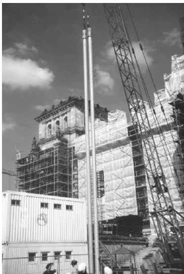
FIGURE 11: Double pipe installation
