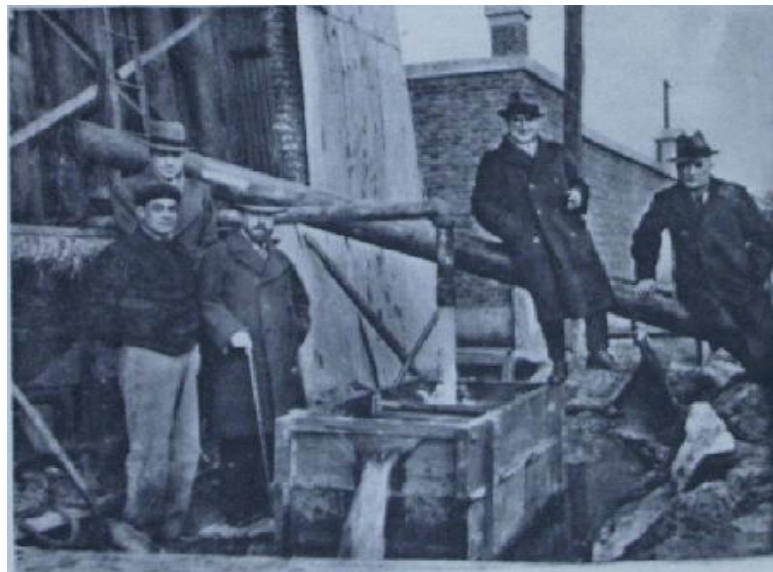
FIGURE 4: Pumping test in situ of first geothermal well in 1936
