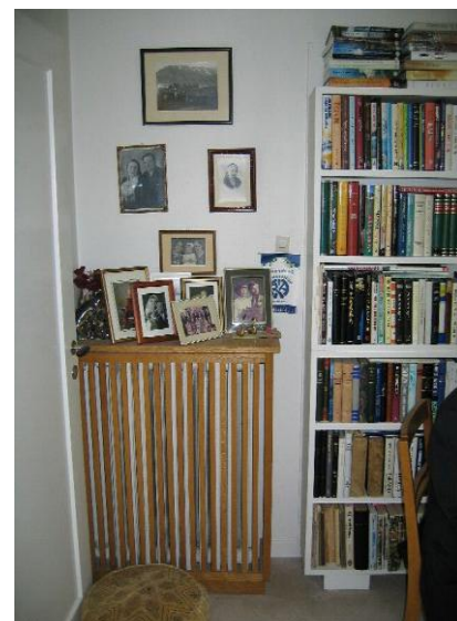
FIGURE 7: Wood covered radiator
