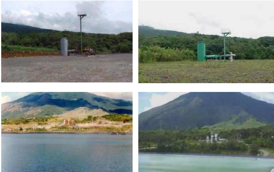
FIGURE 6: Work site before and after recovery activities
