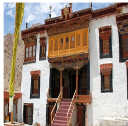
FIGURE 1: A house in Chumathang
