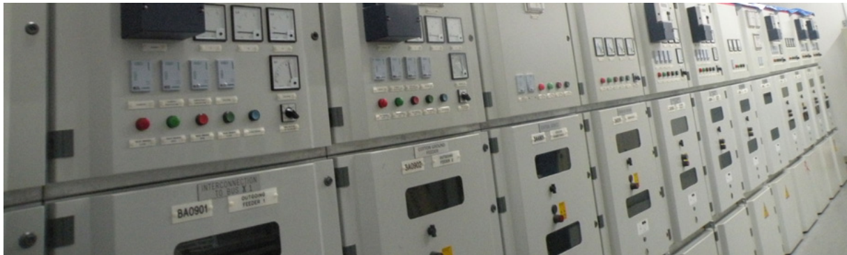
FIGURE 22: Substation switchgear
