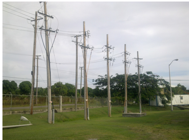
FIGURE 23: Five 11 kV feeders leaving PPS via overhead lines
