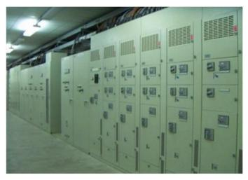
FIGURE 12: Motor control centres (MCC) at Olkaria II power plant
