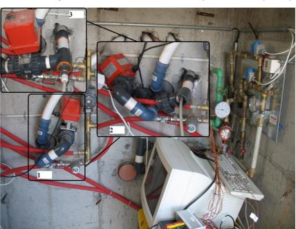
FIGURE 21: Rubber pipe installation steps using pot drainage pipe
