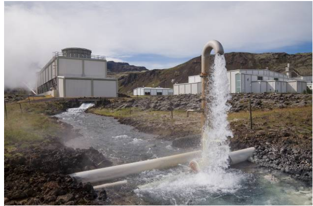
FIGURE 5: Condensate water from the Nesjavellir power plant and well SV-3 (in the distance)
