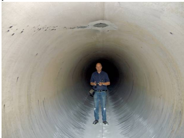
FIGURE 6: Inside the retention tank
