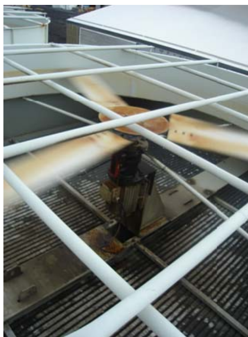
FIGURE 14: Svartsengi plant modified gear coupled cooling fan
