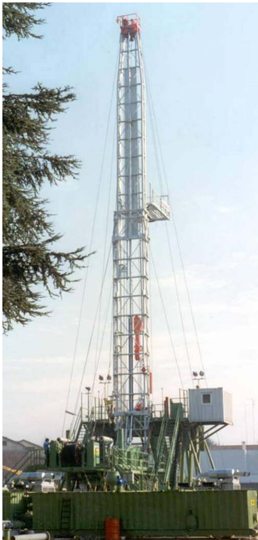
FIGURE 8: Drilling rig at Tendaho
