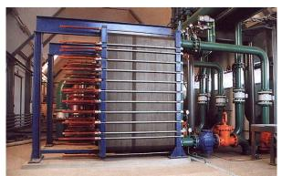
FIGURE 4.10: Geothermal base load plant, Banska Nizna – plate heat exchangers (photo T. Kliszcz)
