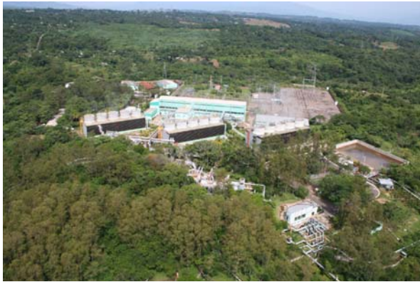
FIGURE 6: Ahuachapán power plant
