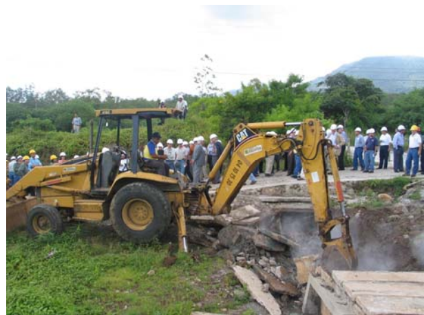
FIGURE 12: Decommissioning of the canal to the sea in August 2004
