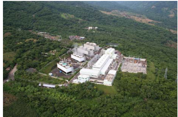
FIGURE 7: Berlín power plant
