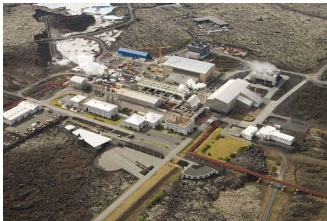
FIGURE 1: A current view of the Svartsengi power plant
