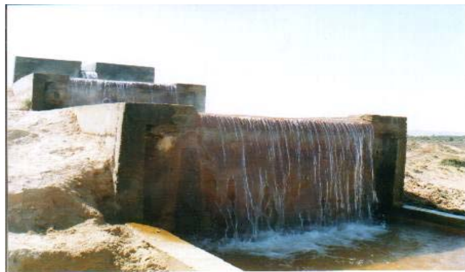
FIGURE 3: The water cooling system (Cascade of Oum Elfareth, Kebili area)
