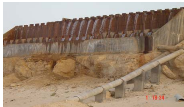
FIGURE 4: The water cooling system (Cascade of Oum Somaa, Kebili area)
