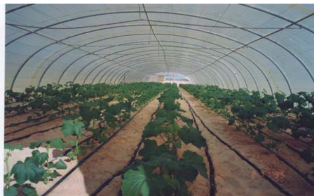
FIGURE 10: The heating system
