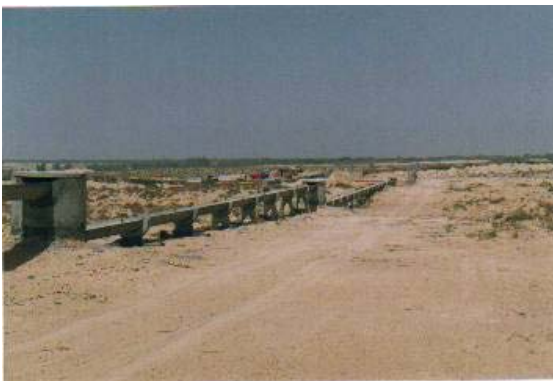
FIGURE 6: The concrete canalization for oasis irrigation (Bazma project, Kebili area)
