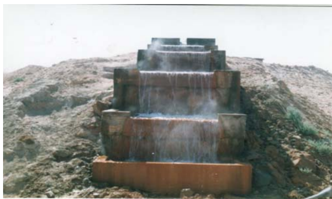
Figure 2: The water-cooling system (Cascade of Oum Elfareth).
