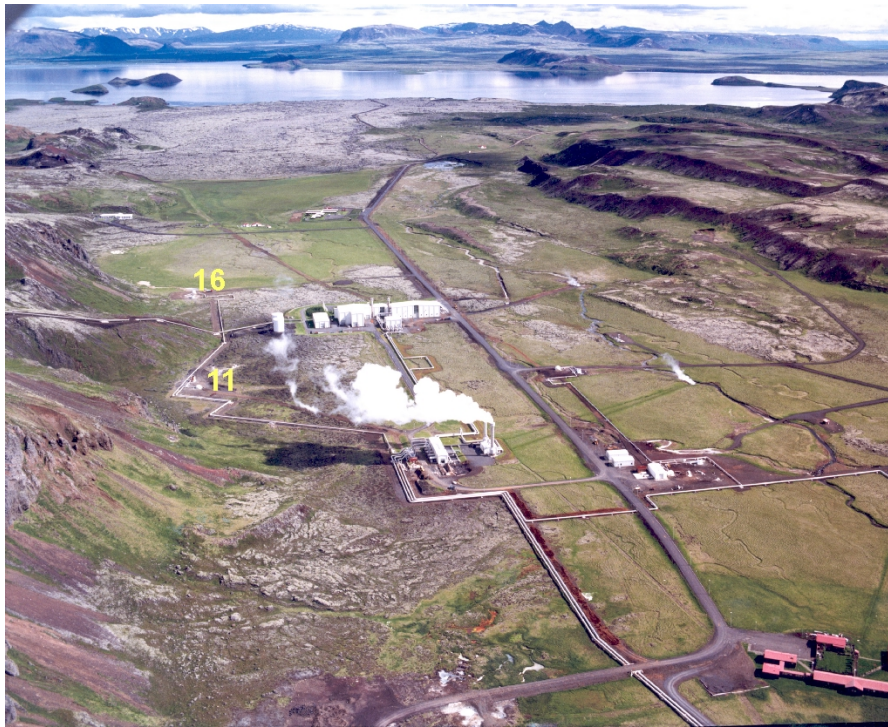
Figure 9. The Nesjavellir power plant was built just east of wells no.11 and 16 (photo by Emil Þór)
