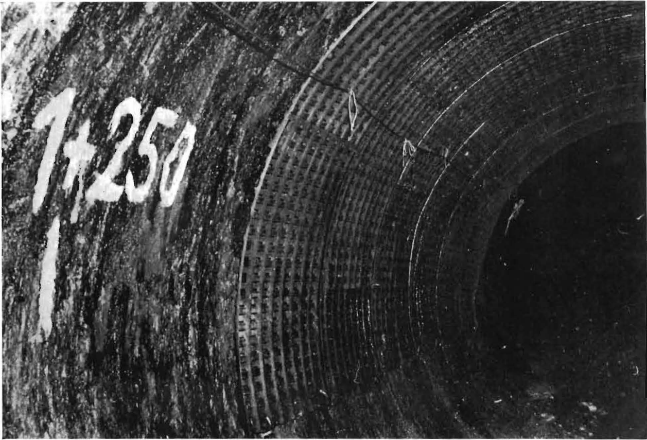
Fig. 27 Securing of the ring in the Oker-Grane-Gallery
