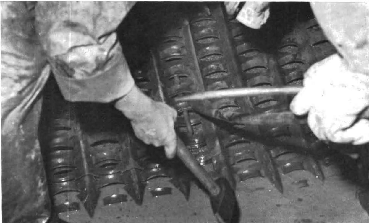
Fig. 24 Locking of the sheets
