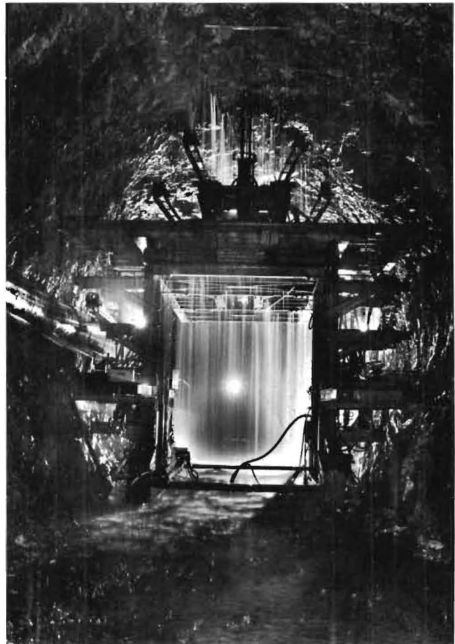
Val S-charl headrace tunnel Engadine hydro plant, Switzerland. Heavy rain from very permeable dolomite, tunnel diameter is 5.70 m
