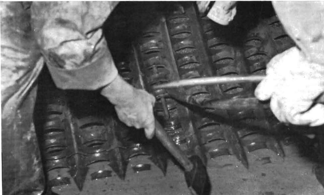
Fig. 24 Locking of the sheets
