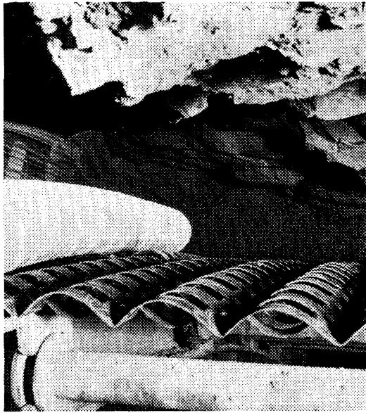
Fig. 5 View of cavity between the sheets and the rock face. When fitting the sheets a concrete of stiff-plastic consistency is poured at the same time. On the left is a flexible concrete supply pipe.
