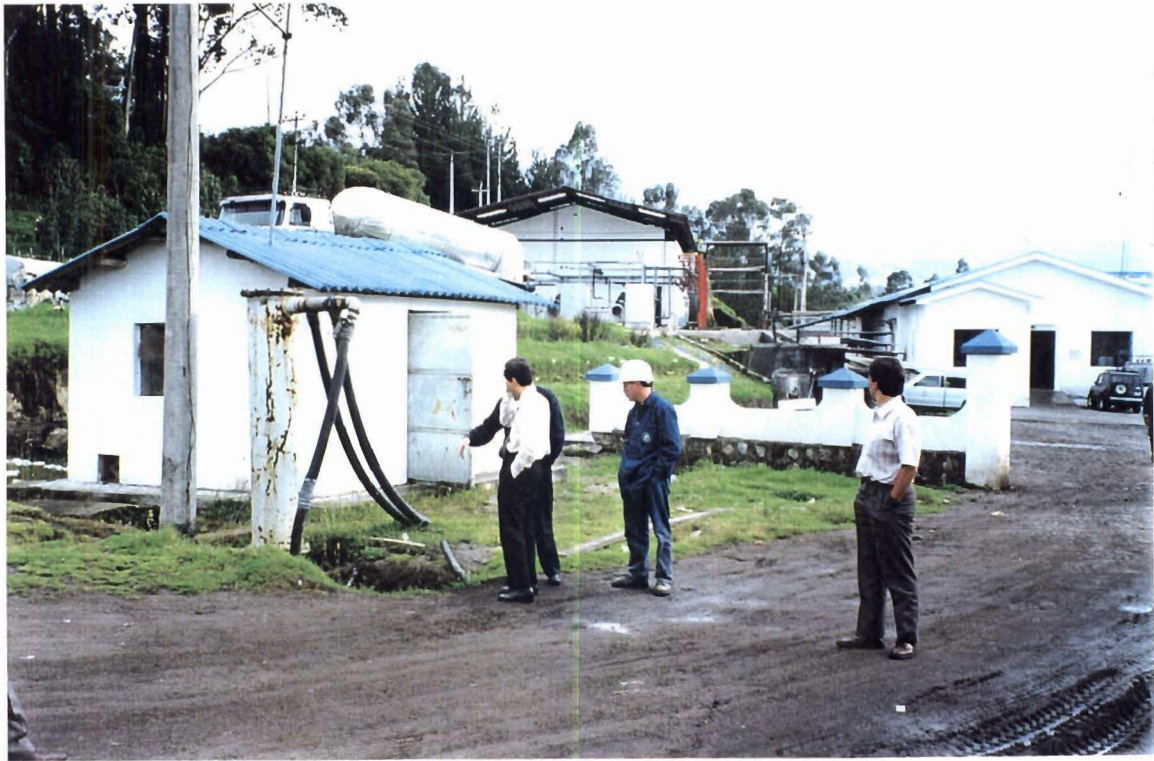
Picture 3. The gas header before the second booster pump. Plant and office in background.
