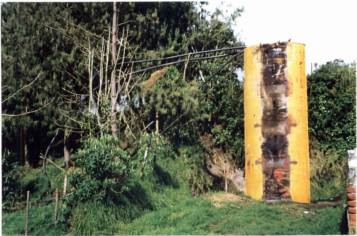
Picture 11. Steel separator on well Margarita by the plant.
