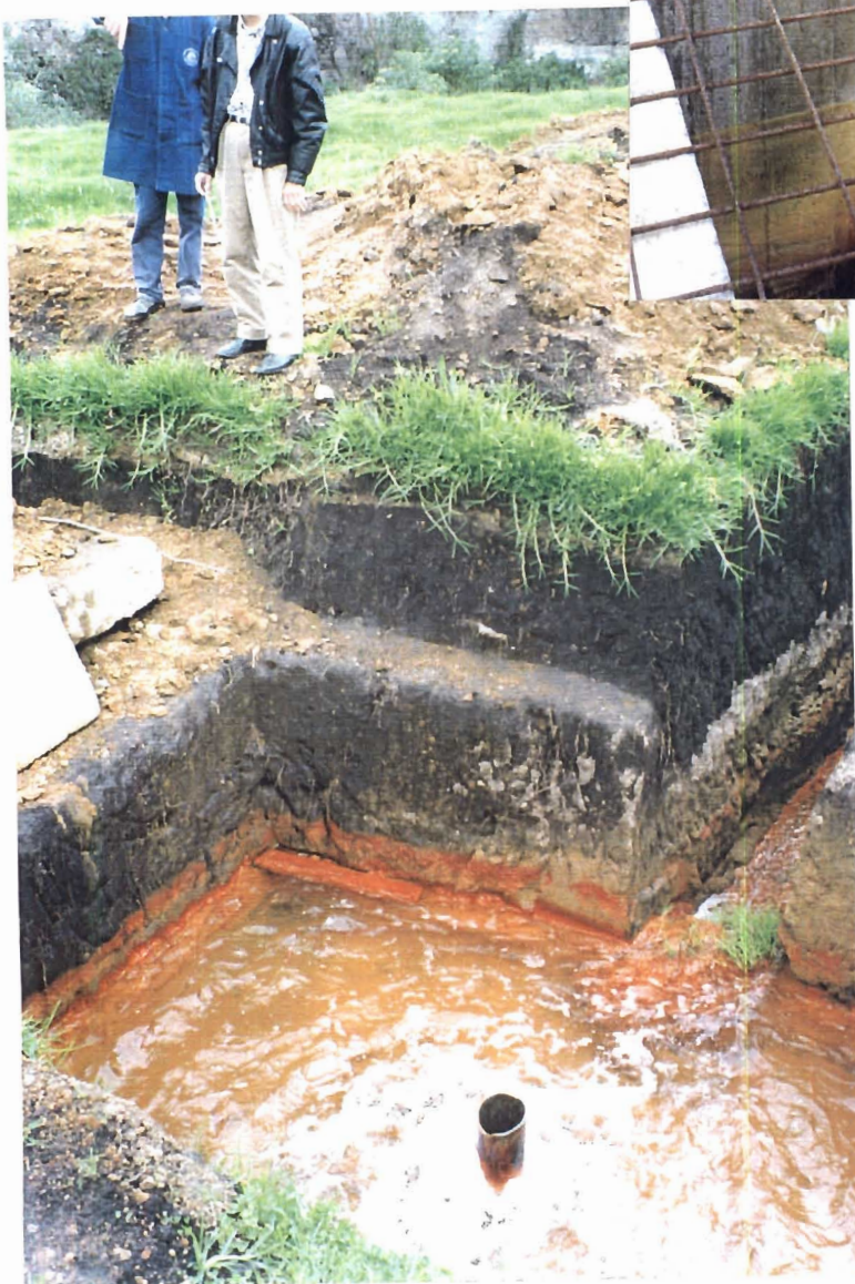
Picture 8. Tatatambo Alto note uncontrolled gas outflow through the annulus.
