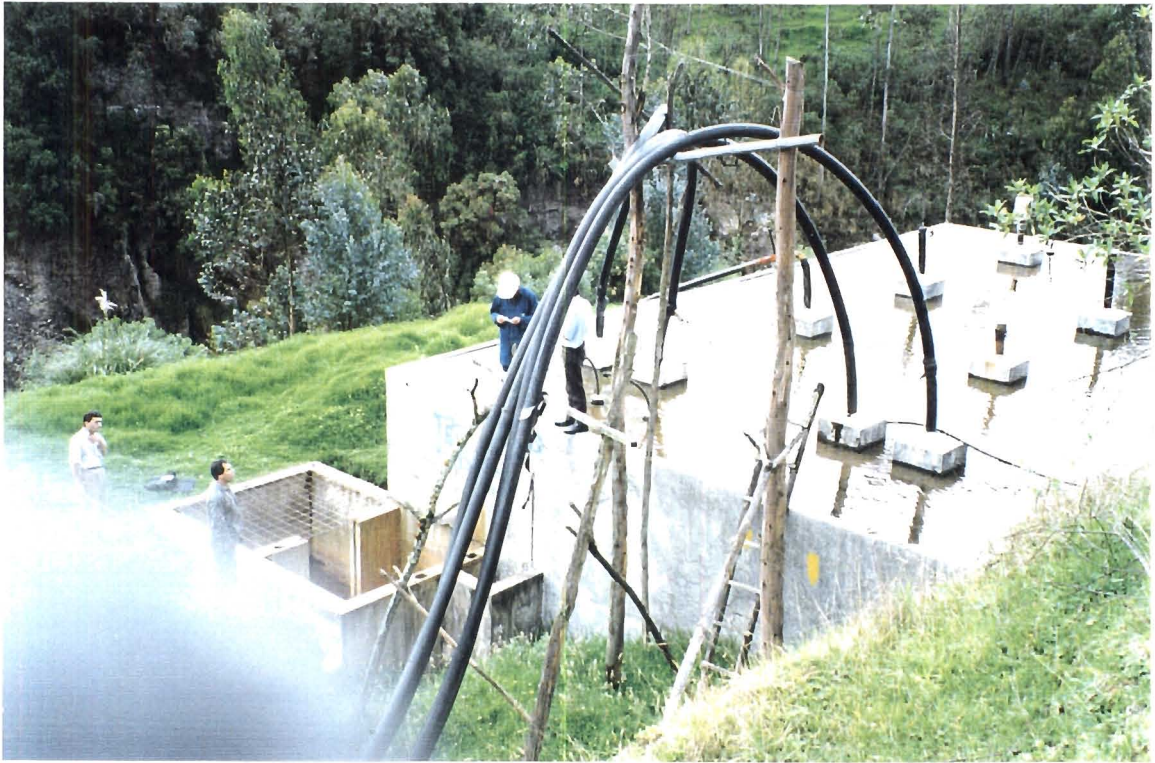
Picture 5. The gas separator at San Guillermo with water outflow box on the corner.
