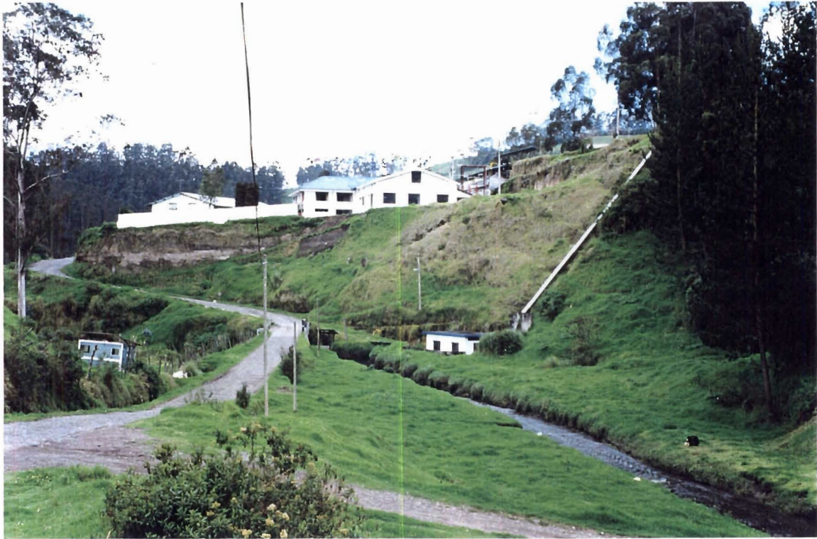
Picture 1. Agua y Gas de Sillunchi SA. The plants mini-hydro 125 kW is by the river.
